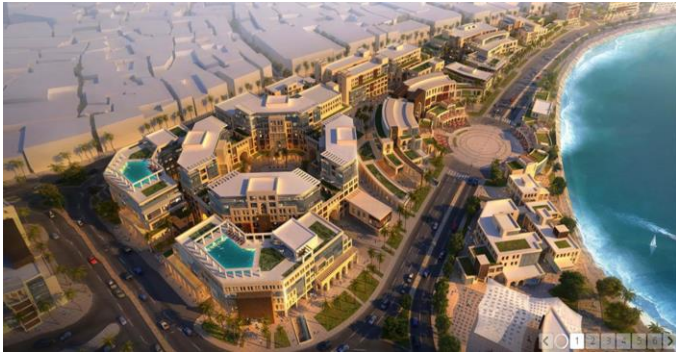
Deira Enrichment Development (2019 - Ongoing) Deira, Dubai Plot 1, 2, 3, 9, 11 & 13 3000+ Residential Units
