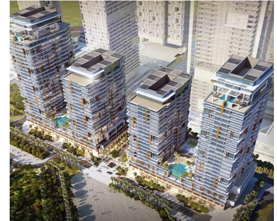
Kifaf Development - Phase 1 (2020) Al Kifaf, Dubai Luxurious Residential Development 2500+ Residential Units
