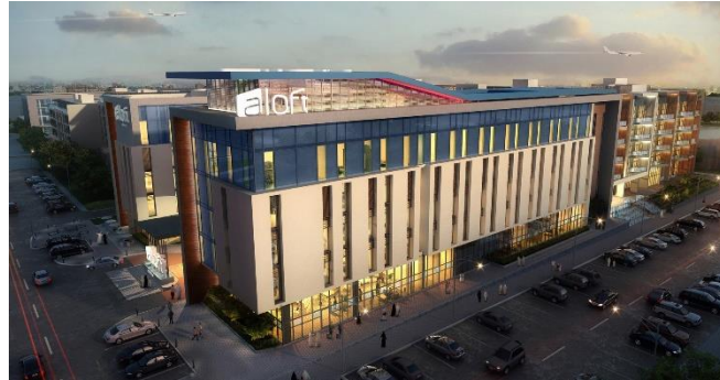
Aloft Hotel & Element Hotel Apartments (2020) Al Garhoud, Dubai B+G+4+R 518 Guestrooms
